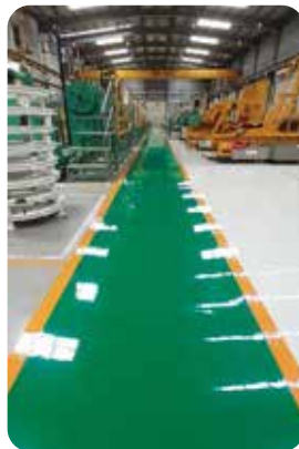
PT. CG Power Plant
